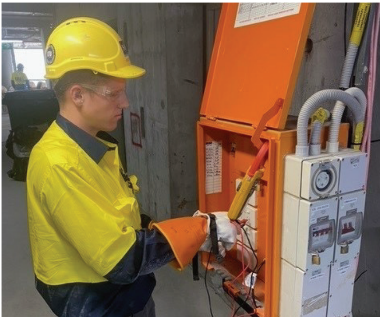
Figure 1: Completing electrical work safely.
