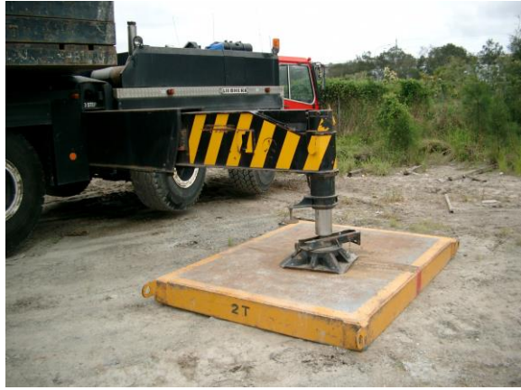
Figure 8 - Crane outrigger foot on bog mat
