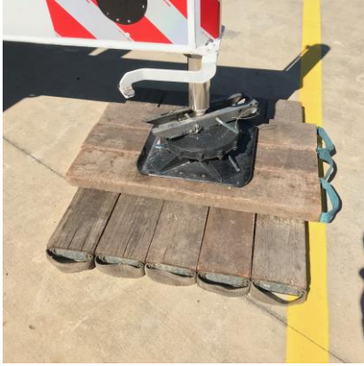
Figure 7 - Crane outrigger foot on timbers
