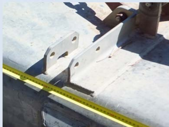
Image 5: Steel plates welded to slasher deck for pinning props
